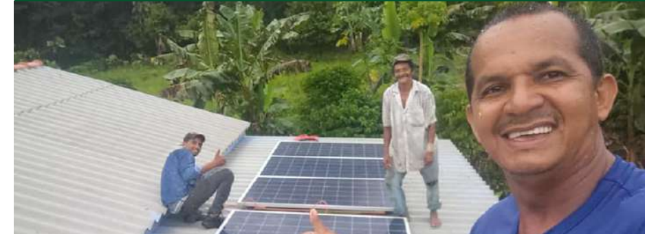
Installation of solar panels
